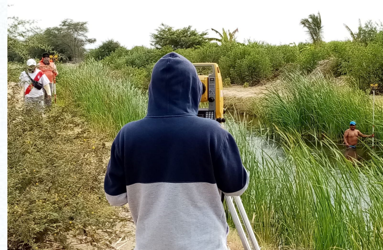
Hired Sub-Consultant (Luis Solis + Team) Conducting Topographic Land Survey in Las Mercedes KM11 to be used in the Clean Water Solution Design. (2022-09-20)
